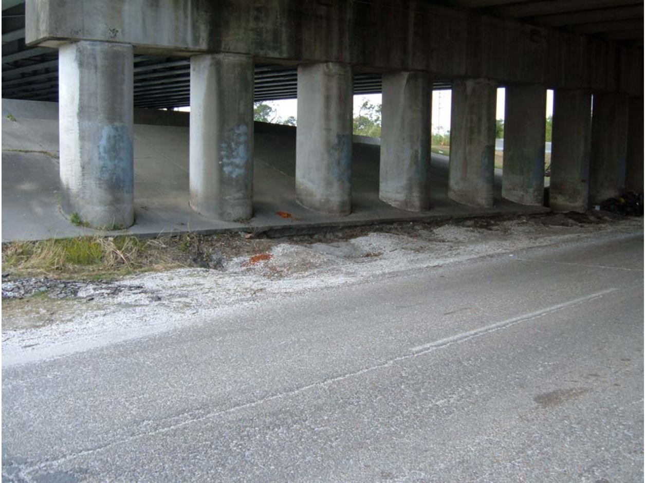
Figure 1-75. Scour between columns below low pump station wall at OP#7. Low wall is at top of slope behind concrete columns.
