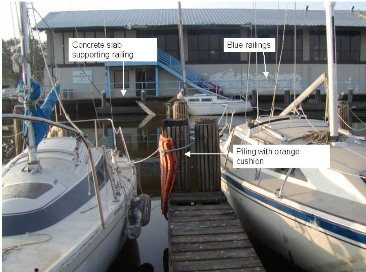
Figure 1-8. Railings, pilings, and other features near Municipal Yacht Harbor Building. Looking south
