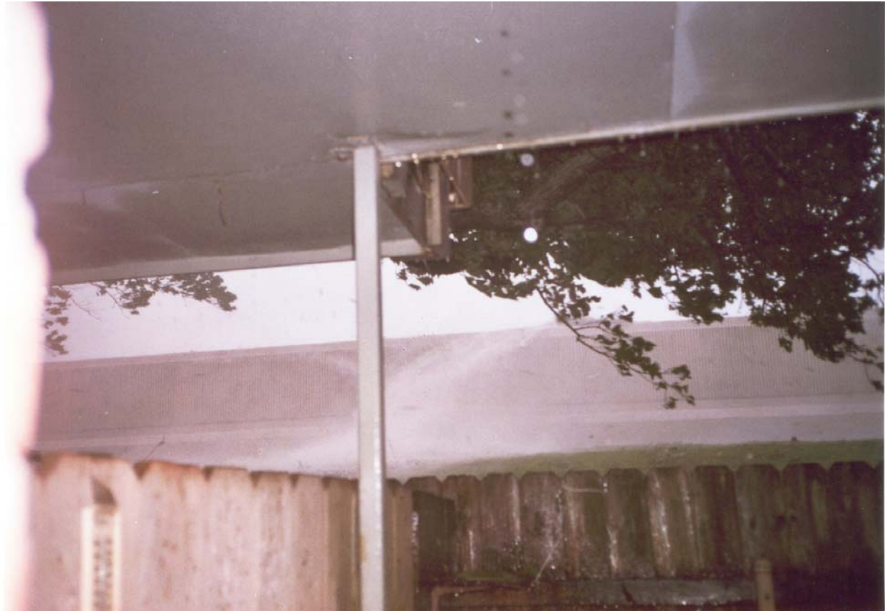
Figure 1-87. Wave spray or splash (left of tree limb) at west wall of 17th Street Canal north of Veterans Blvd and 1.0 mile south of Hammond Hwy. The individual who took this picture stated that the tree limb obscures the crest of a wave.
