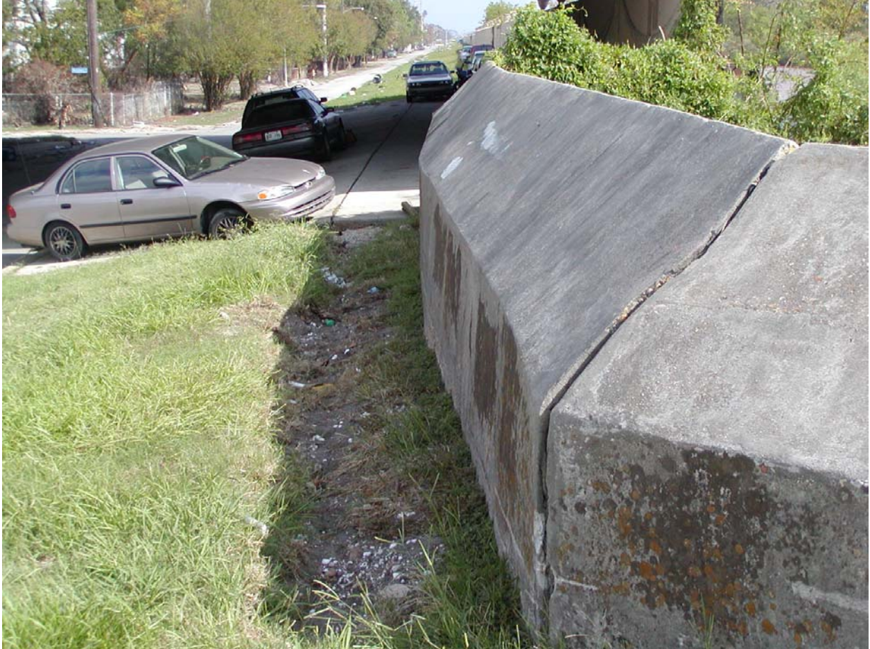
Figure 1-78. Scour below OP#7 low pump station wall on west side. Note that fall distance and scour is greater on this side than on the east side. Note floodwall in background that is about 4.3 ft higher.
