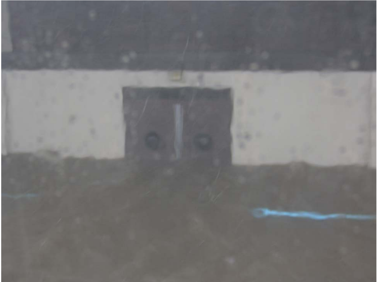
Figure1-14. Picture DSC02240.JPG taken at 0826:32 (CDT) on 8/29/05, elevation 9.1 ft. Looking south. Water level at upper rail.
