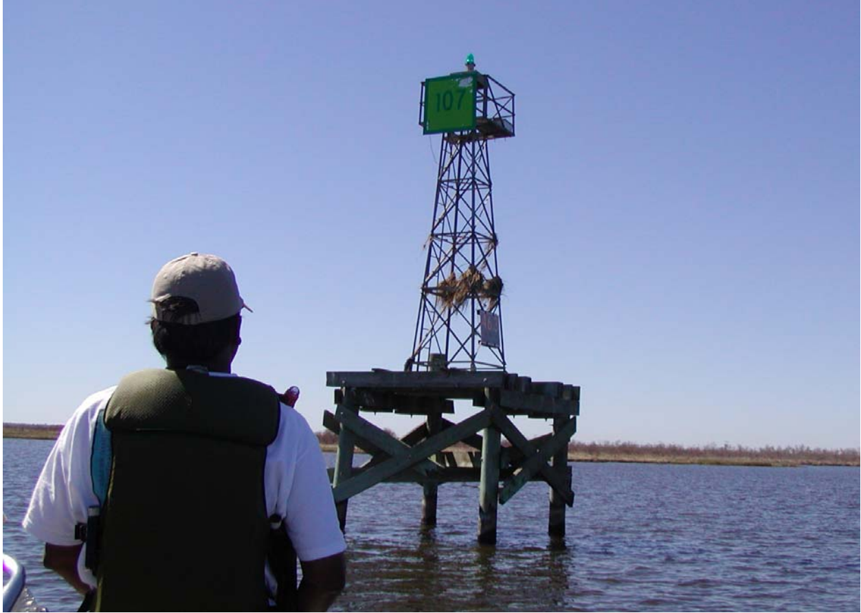
Figure 1-102. LA 1155 on MRGO. Debris on tower.
