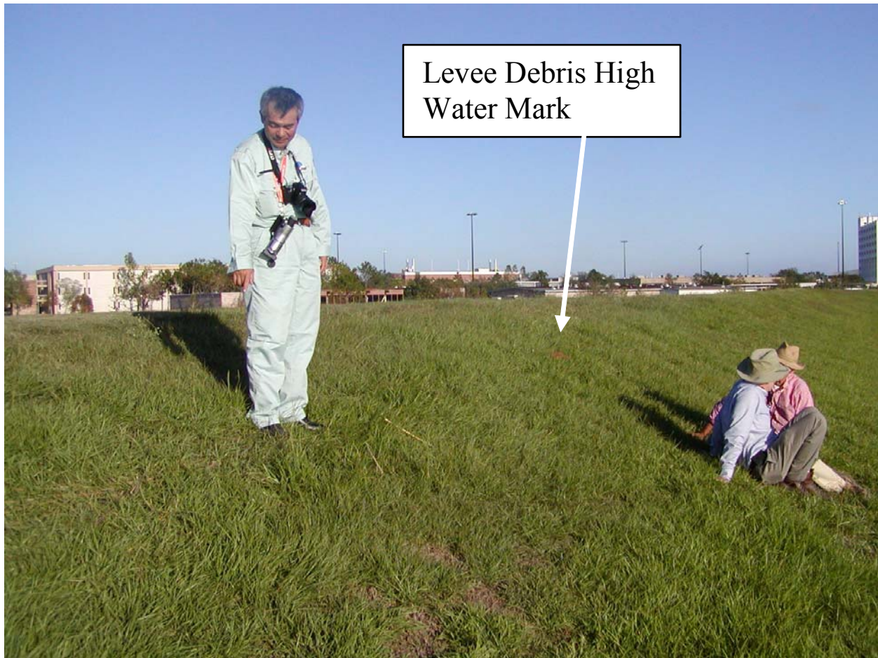
Figure 1-96. Debris high water mark LA 1022 on east levee of London Avenue Canal north of Leon C Simon Drive.
