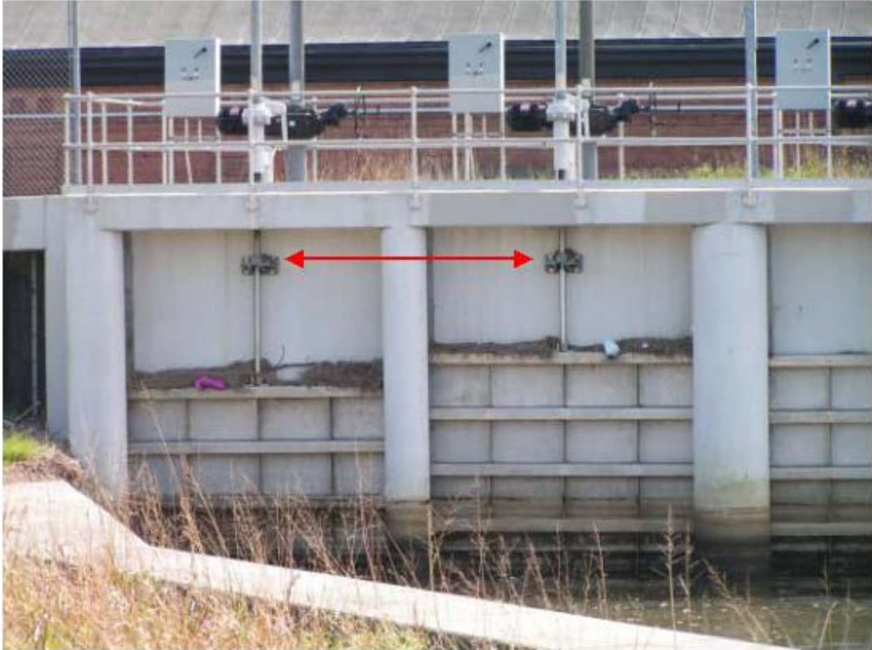
Figure 1-85. Debris high water mark at top of brackets holding gate rods on east side of discharge area.
