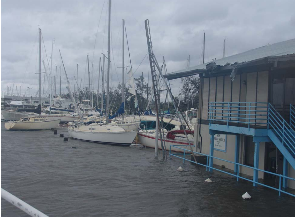
Figure 1-17. Picture DSC02262.JPG taken at 1538:44 (CDT) on 8/29/05, elevation 6.5 ft. Looking east-southeast. From left to right vertical posts, water level is 0.7, 0.8, 0.8, 0.7, and 0.6 ft below the center of the lower rail.
