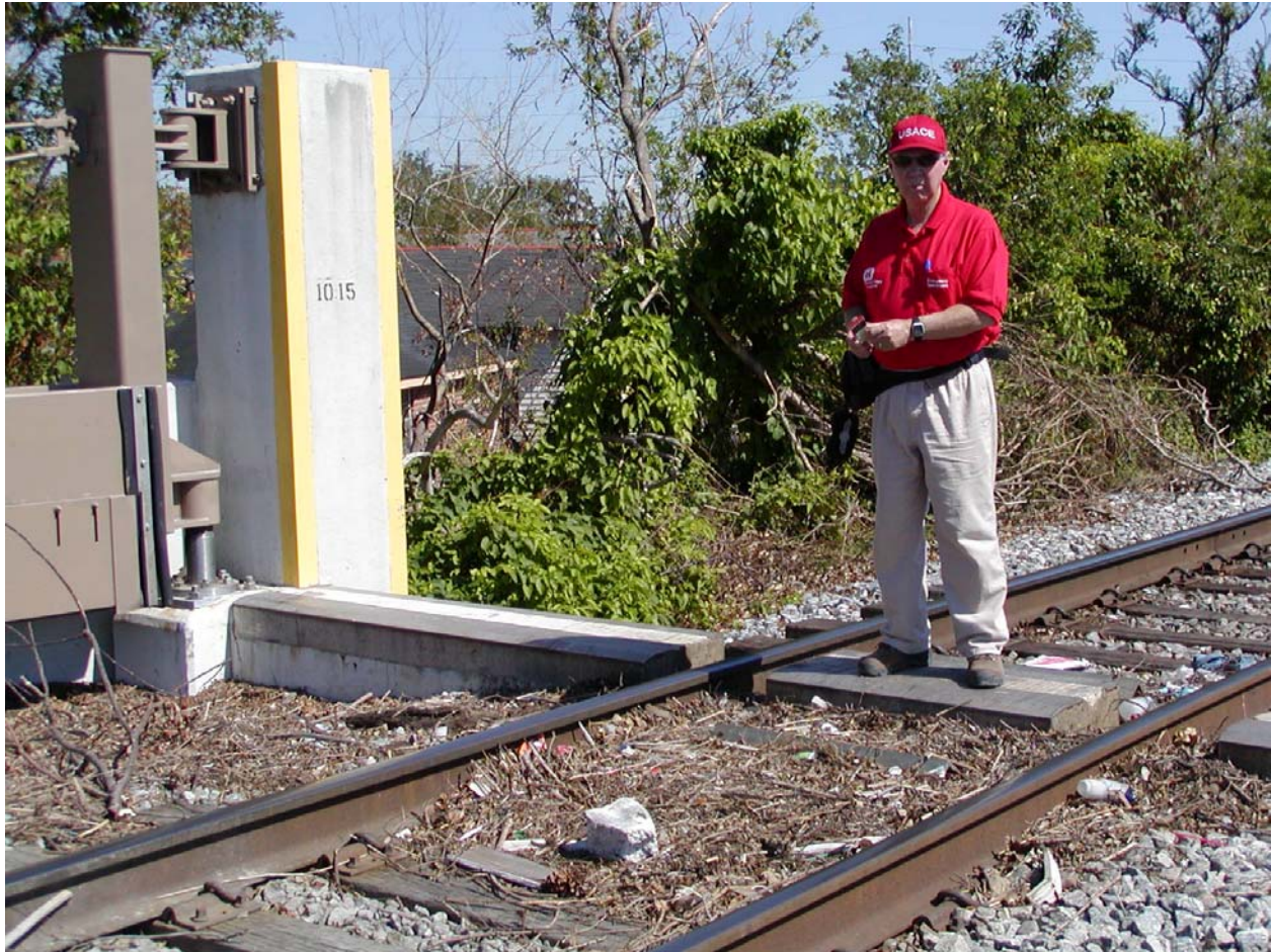
Figure 1-97. East floodgate at OP#3 at south end of London Avenue Canal. High water mark LA 1227 at top of railroad ties.
