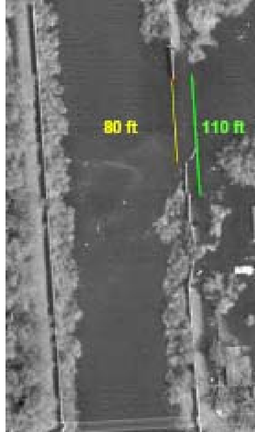
(b) South breach at Mirabeau Avenue
