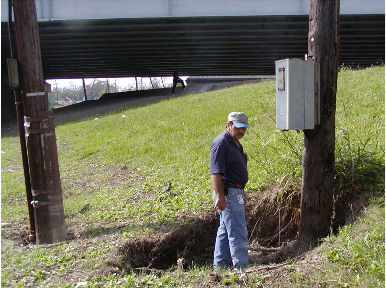
Figure 1-76. Scour around power pole below earth levee on east side of Orleans Ave Canal.
