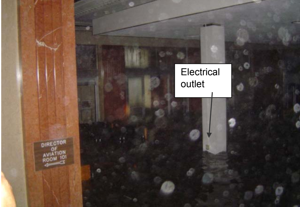
Figure 1-44. Time = 10:56 AM, APH-08. Column in terminal building lobby.
