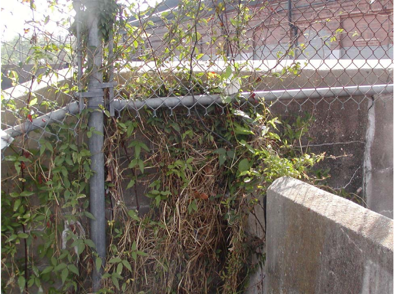
Figure 1-79. Debris caught in vegetation showing flow over low wall at OP#7. About 6" above low wall on west side.
