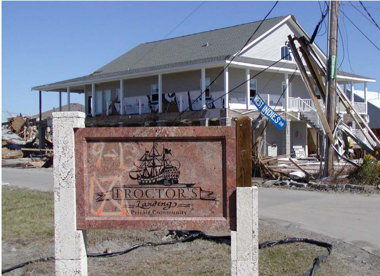
Figure 1-103. Home in Shell Beach containing high water mark LA 1087 at 31" above second level floor.
