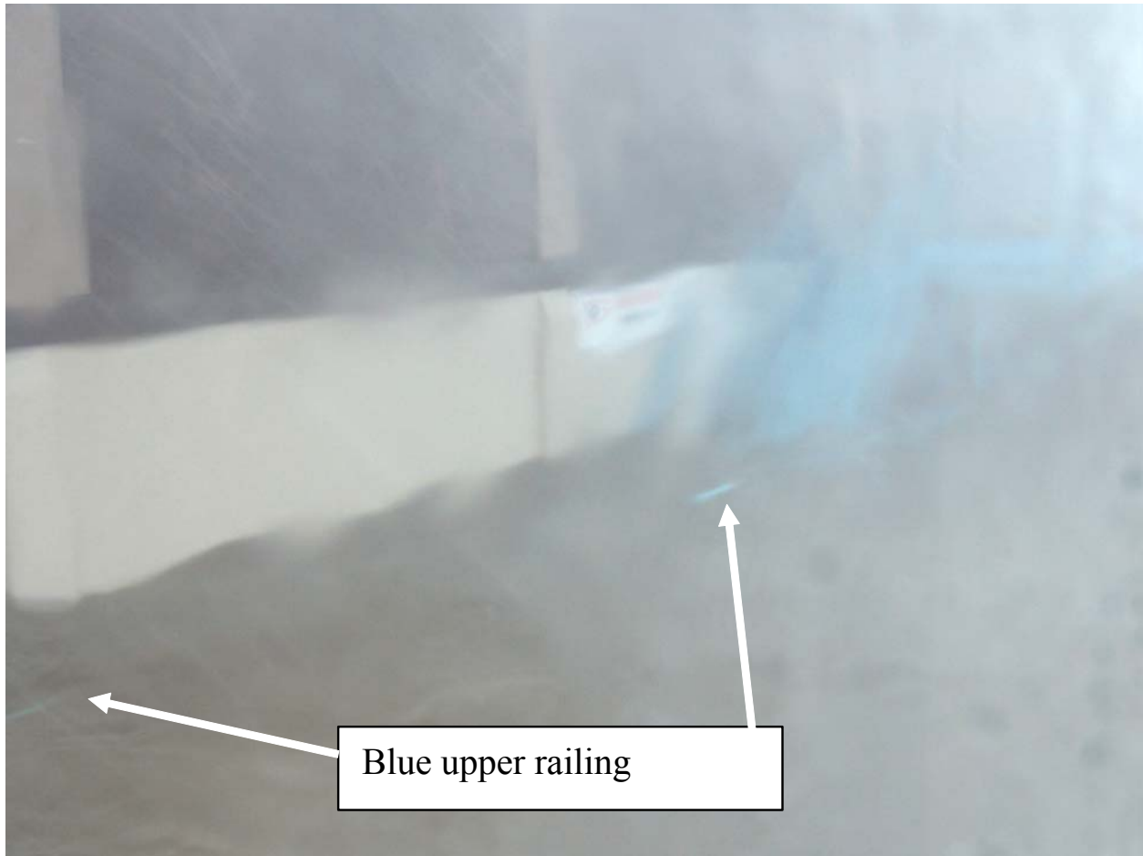
Figure 1-15. Picture DSC02241.JPG taken at 0826:36 (CDT) on 8/29/05, elevation 9.1 ft. Looking south. Water level at upper rail. Brightness and contrast adjusted.
