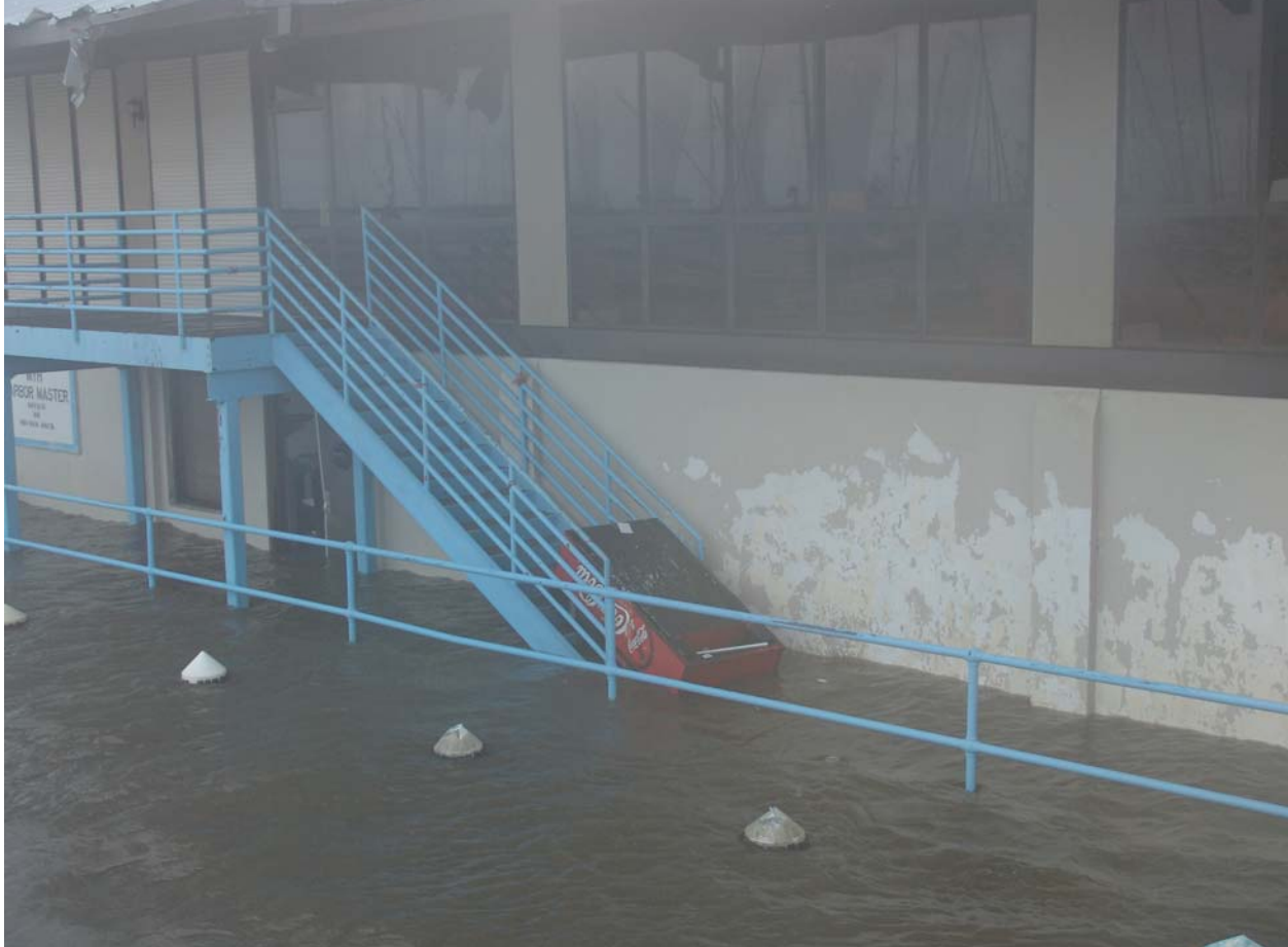
Figure 1-18. Picture DSC02263.JPG taken at 1538:54 (CDT) on 8/29/05, elevation 6.5 ft. Looking southeast. From left to right, water level is 0.5, 0.7, 0.7, and 0.9 ft below the center of the lower rail.
