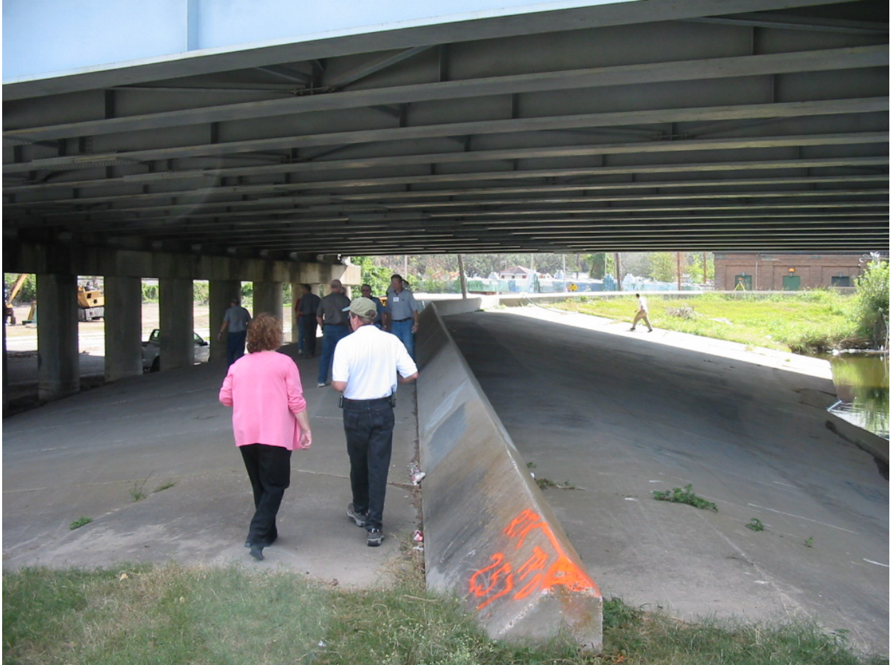
Figure 1-73. Low wall that connects to OP#7 at Orleans Avenue Canal looking south-southeast standing on earth levee.
