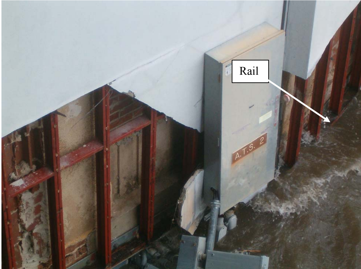
Figure 1-53. Time = 5:30 PM, APH-11. Bottom of horizontal rail to right of electrical panel box on north side of terminal building, east of lobby.
