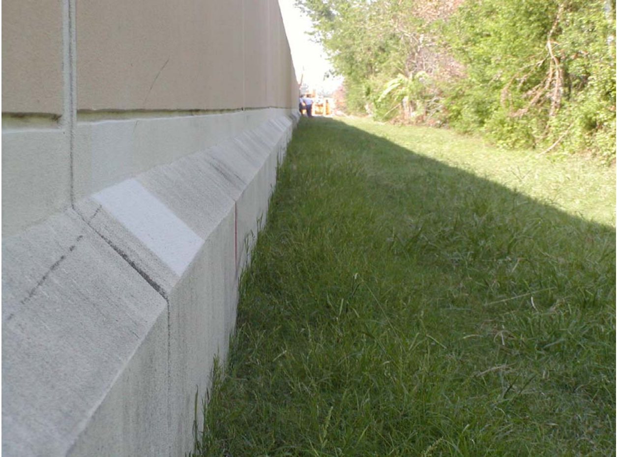
Figure 1-82. Attempt to show possibility of minor scour along west floodwall, south of 17th Street Canal breach.
