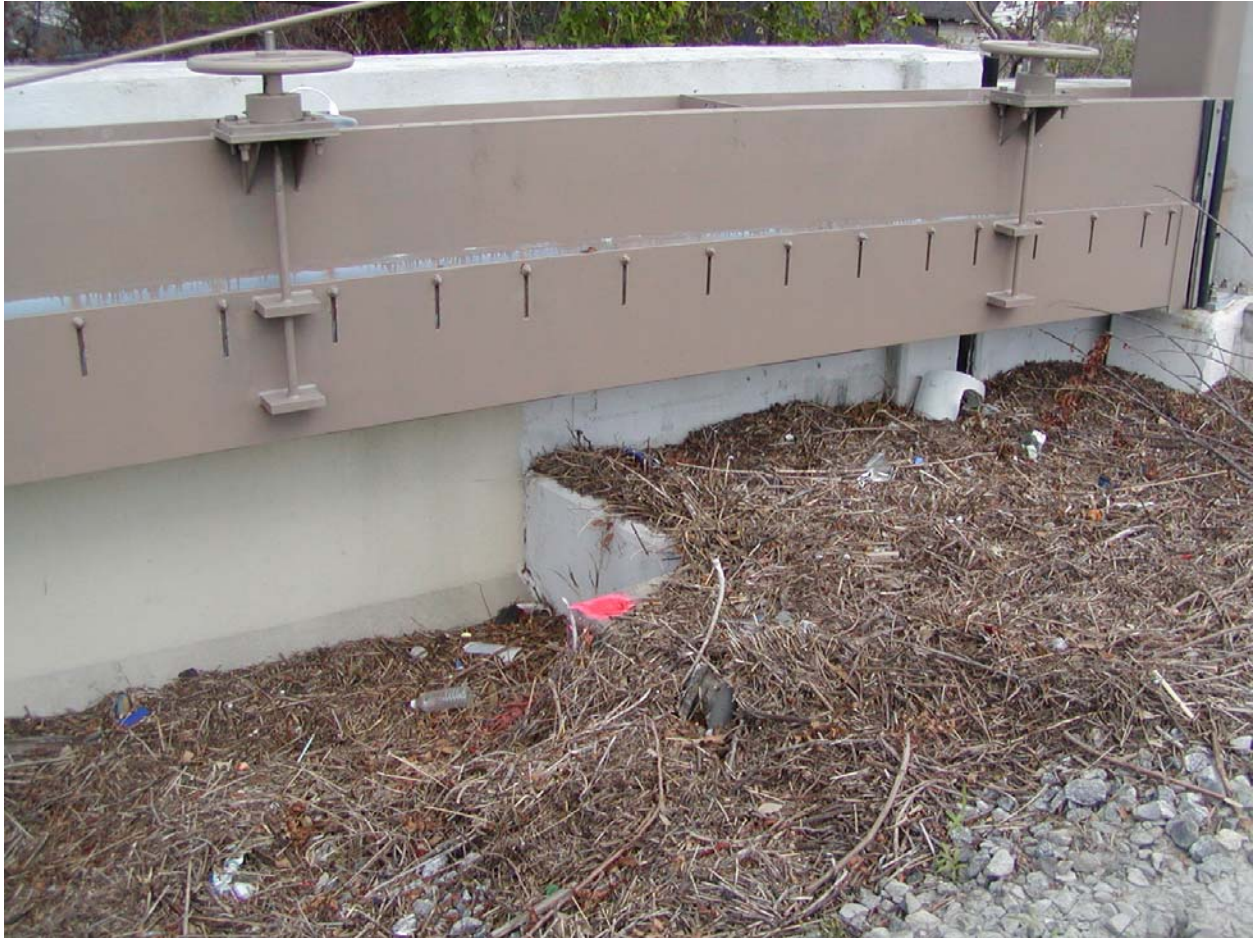
Figure 1-95. East floodgate at OP#3 at south end of London Avenue Canal. High water mark LA 1018 at top of painted concrete wall.
