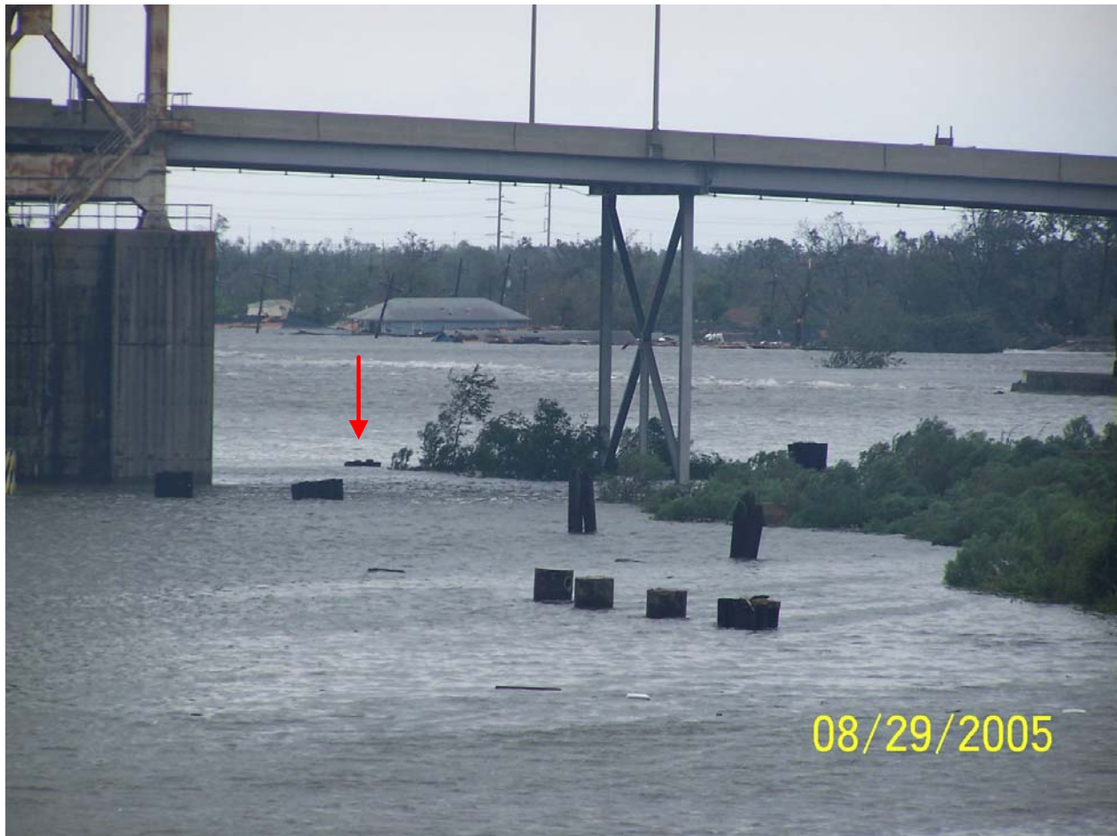
Figure 1-62. Time 3:03 PM, picture 100_0508. Breach on east side of IHNC in background. Looking northeast into Lower Ninth Ward.
