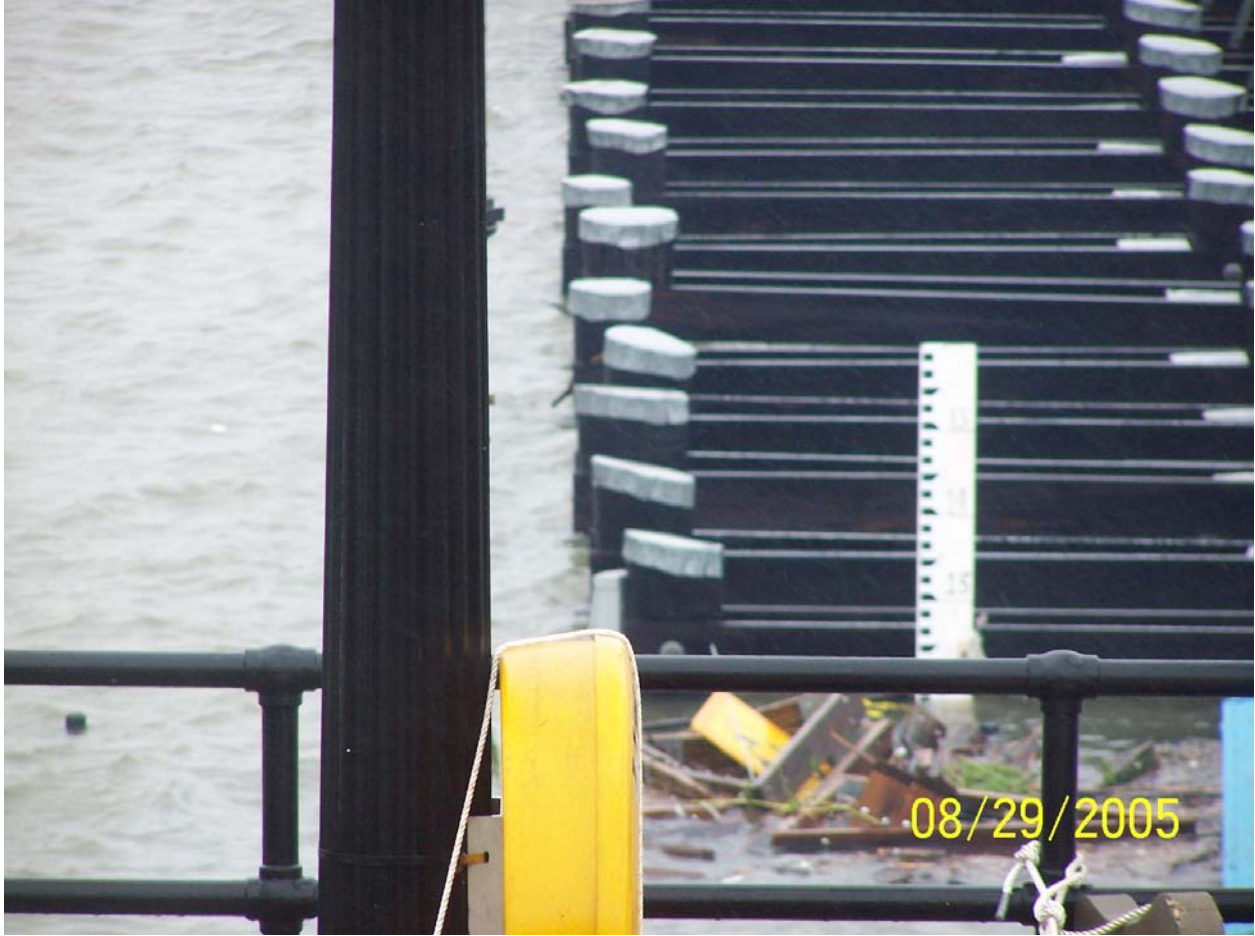
Figure 1-61. Time 11:50, picture 100_0507, looking north.
