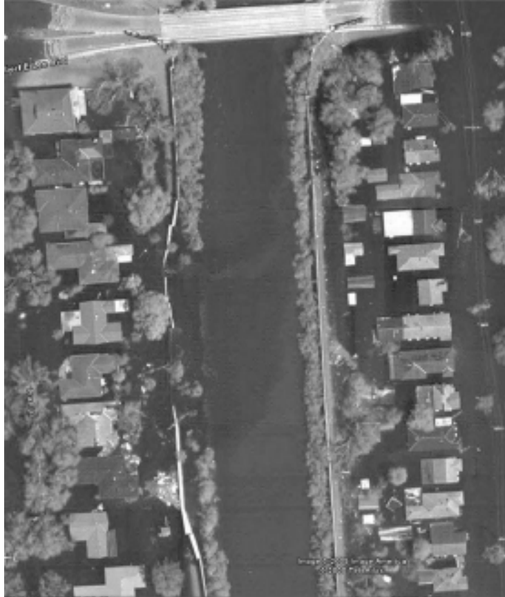
(a) North breach near Robert E. Lee Bridge Figure 11-1. London Avenue Canal breaches
