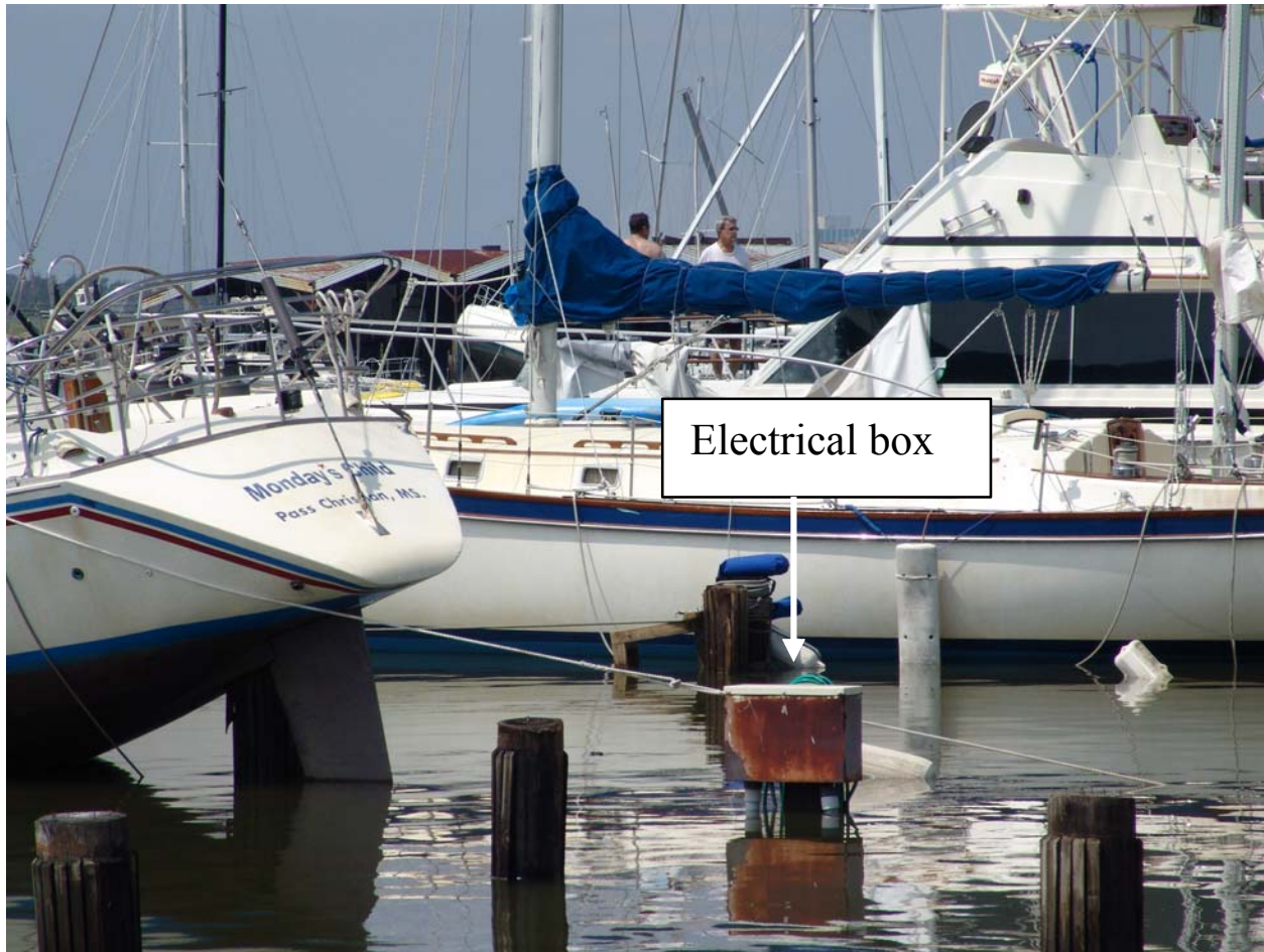
Figure 1-25. Picture DSC02338.JPG taken at 1132 (CDT) on 8/30/05 elevation 4.4 ft. Electrical box at east end of third row of docks
