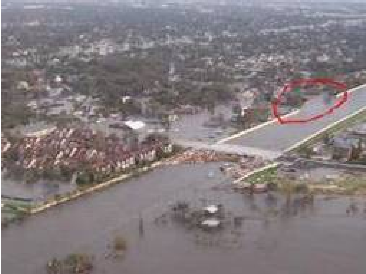
Figure 10-1. 17th Street Canal August 29, 2005. Looking south showing breach and debris impounded against Hammond Highway Bridge
