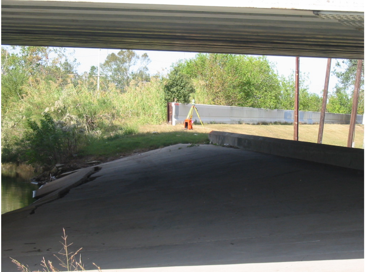
Figure 1-72. Low wall, earth levee, and floodwall in background on east side of Orleans Avenue Canal just north of pump station. Looking northwest.
