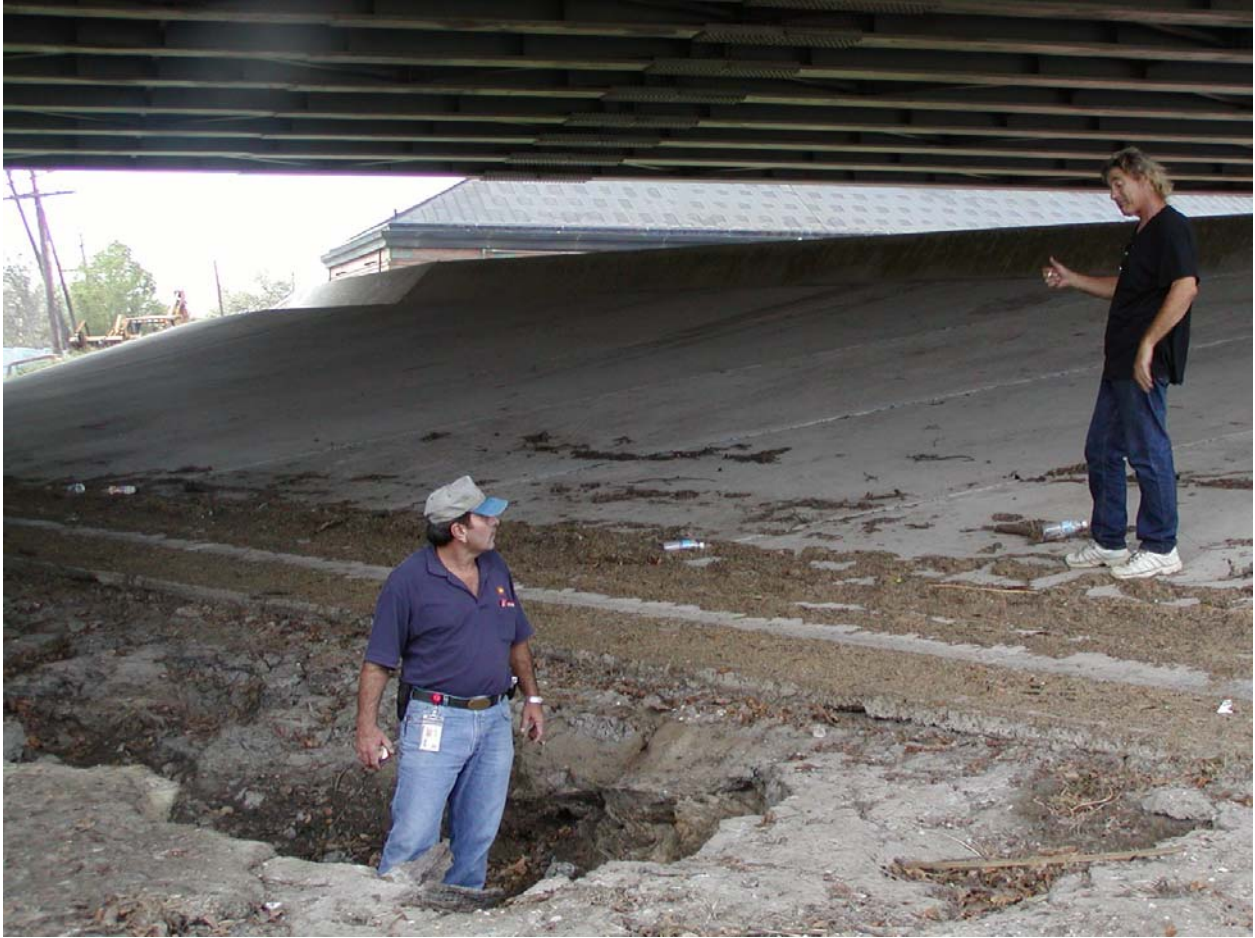
Figure 1-77. Scour below concrete apron that is below low pump station wall on east side of Orleans Ave Canal.
