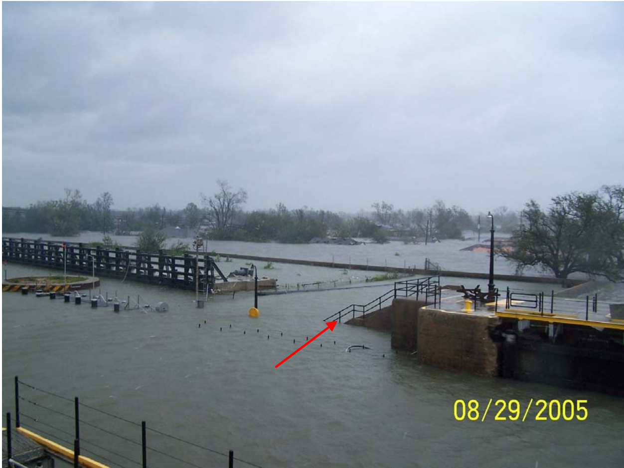
Figure 1-60. Time 11:47, picture 100_0502. Red arrow shows location surveyed. Looking east-northeast into Lower Ninth Ward.
