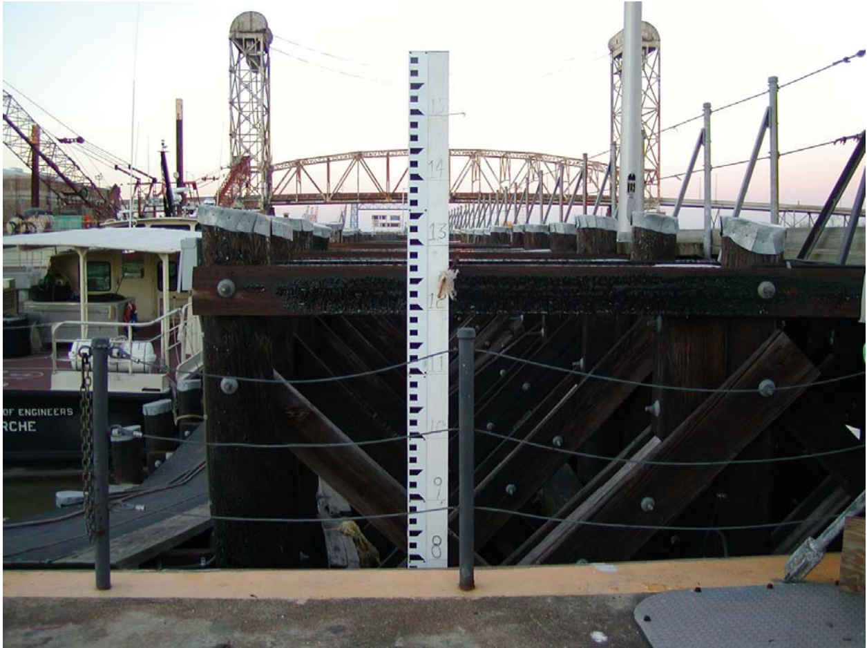
Figure 1-57. Staff gage at IHNC lock. Numbers were far more visible when the lock was visited in October 2005. Picture looking north.
